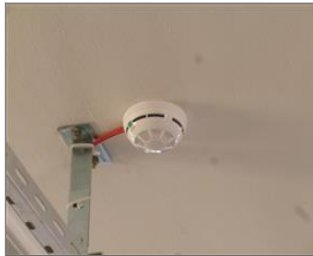
Photo of fire safety equipment Smoke detector.JPG
